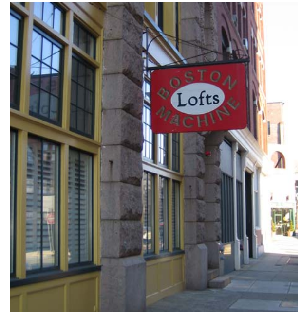
A RECENT DOWNTOWN LOFT CONVERSION
