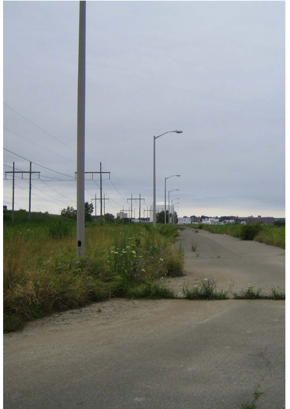
A PUBLIC/PRIVATE PARTNERSHIP IS RESPONSIBLE FOR RELOCATING THE POWER LINES
