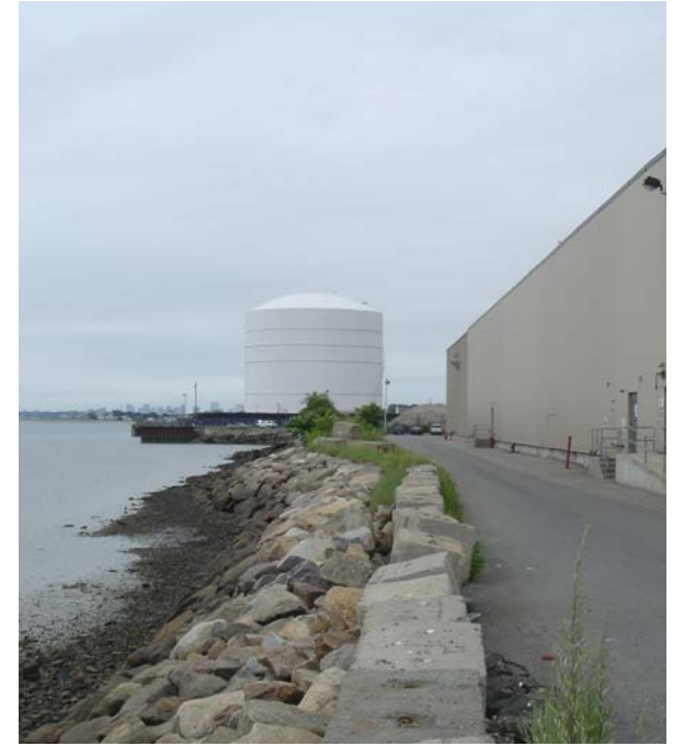
THE LNG TANK AND A DISTRIBUTION FACILITY ARE WINDOWLESS STRUCTURES FEET FROM THE WATER
