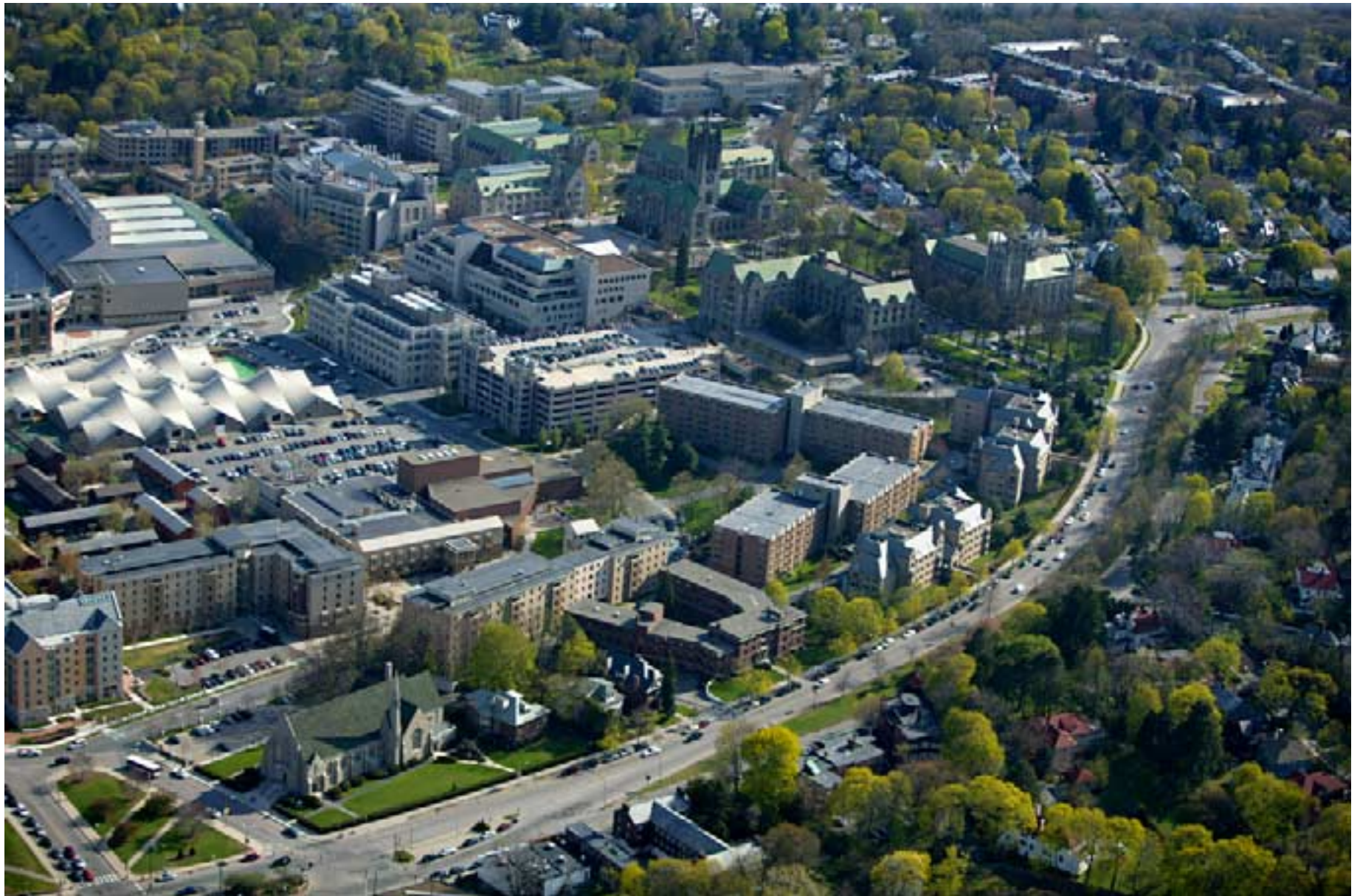
view looking southwest
